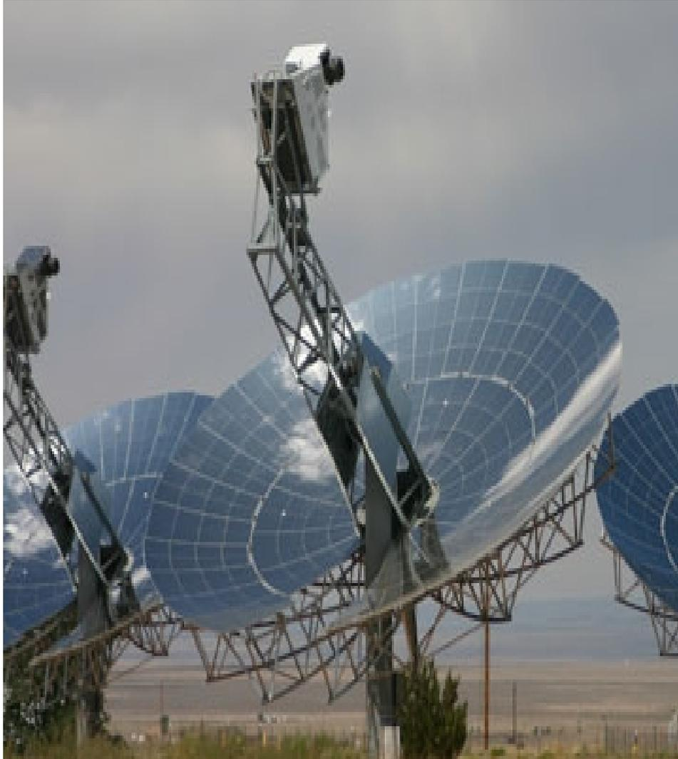
Figura 3 Disco/Motor Stirling. [www.stirlingenergy.com](http://www.stirlingenergy.com)
